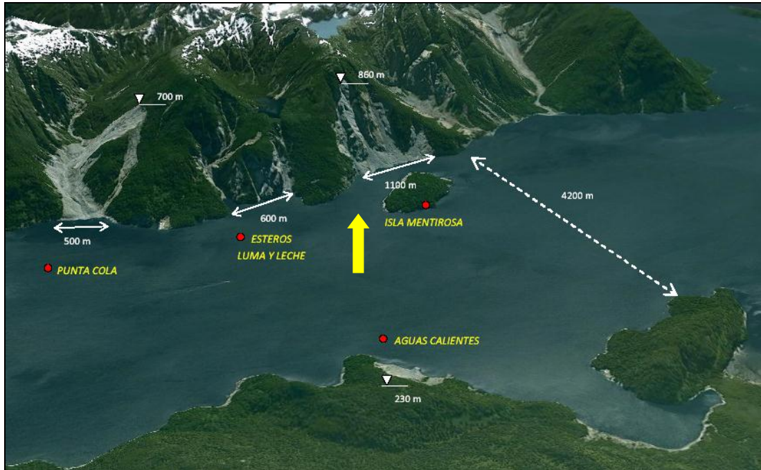
Figure 14: Landslide in front of Isla Mentirosa.
